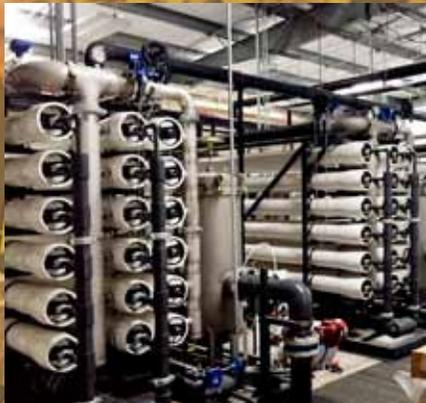
of the new equipment and various site work for the reverse osmosis system is being built on the current water plant site and construction is currently underway. Once the system has completed installation, water quality tests will be performed to determine that target constituents
